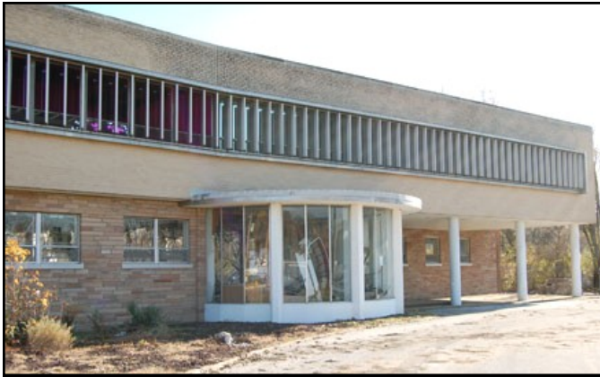
Built in 1957, this sleek modernist building that once housed Universal Match was recently purchased by a neighboring company and is now under demolition
